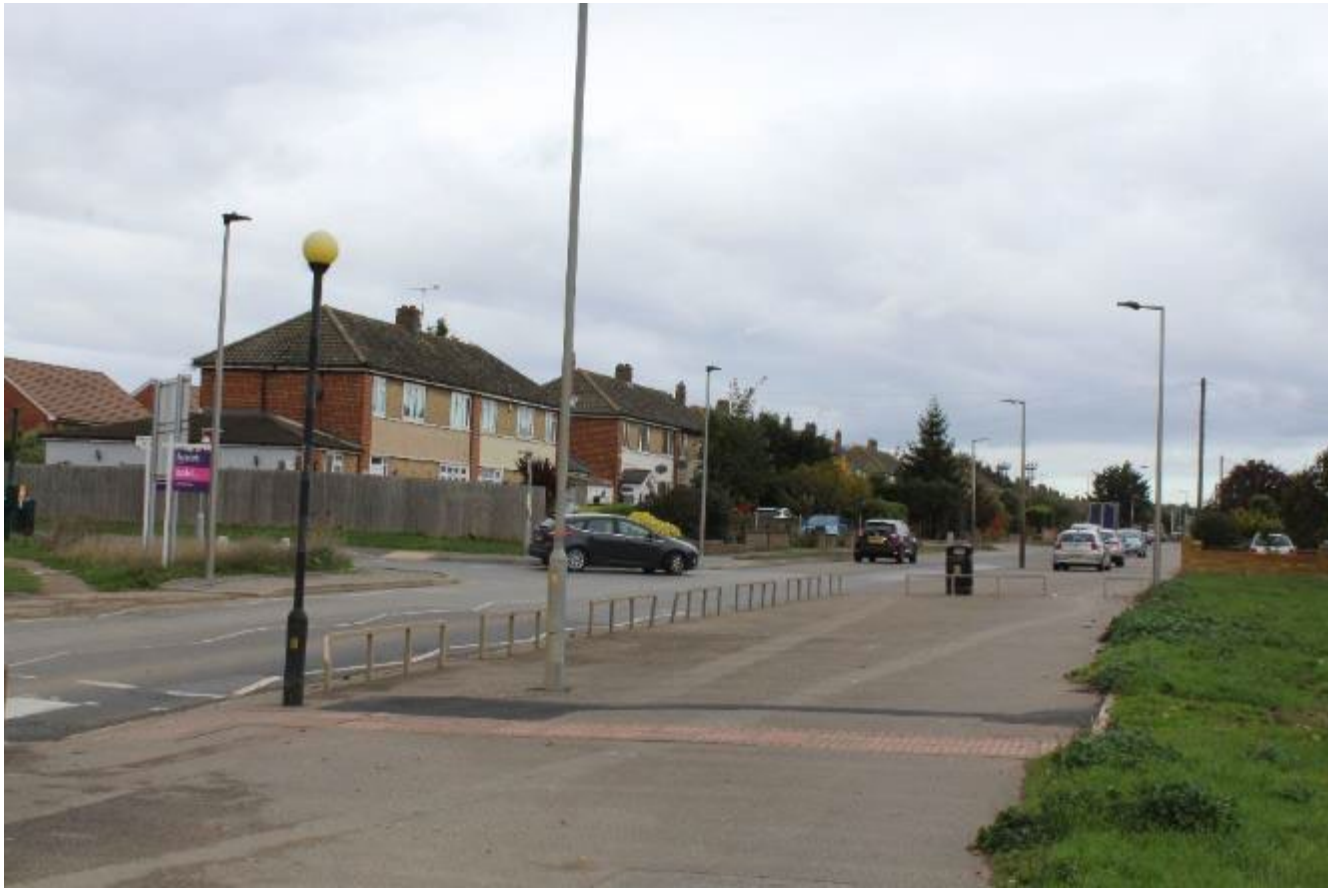
Figure 68: Wide pavements in areas of public realm
